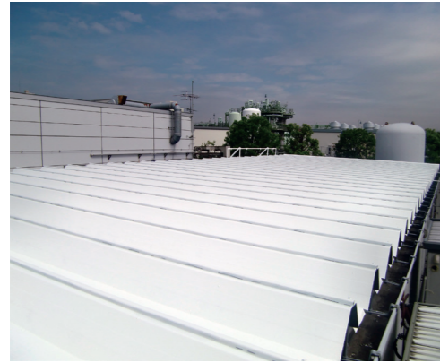
Building Structure Steel-framed structure with colored folded plate roofing.
