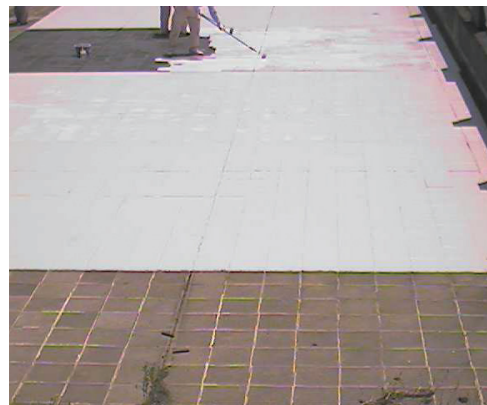
Building Structure RC structure with RC roof covered with waterproof layer and roof mats, with air layer and suspended ceiling.
